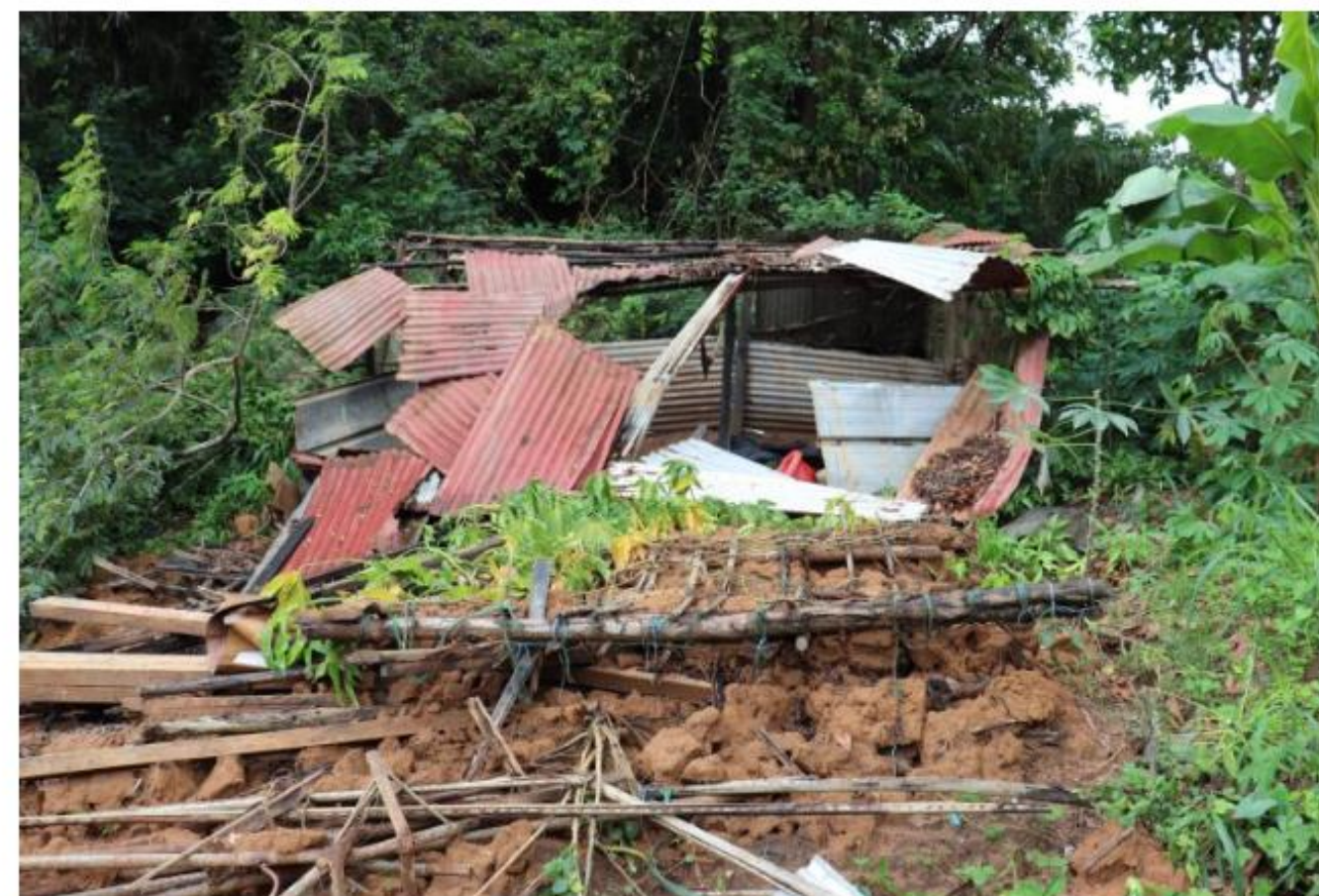
Flood damage in Abidjan, Ivory Coast, June 2022. Photo: ONPC-Côte d'Ivoire
