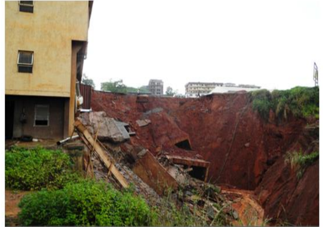
A three-storey building about to be swallowed by gully erosion at Omagbe Estate, Onitsha (Source: News Agency of Nigeria, 2011)
